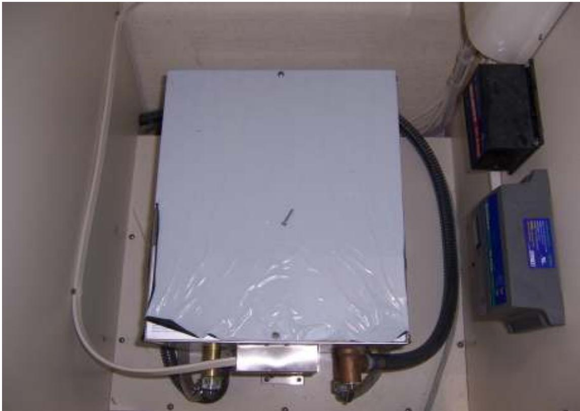
**Galvanic Isolator and Charger on wall by Water Heater**
